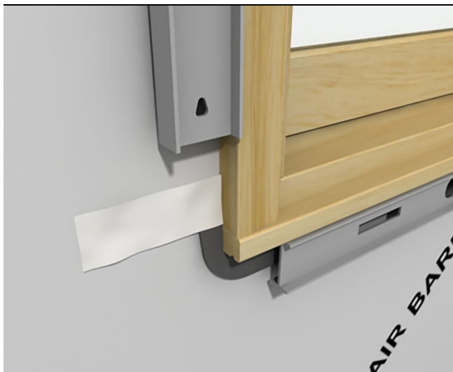
Figure 13 Leveling window, use shims if necessary
