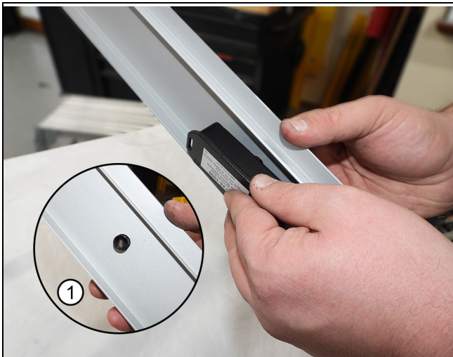
Figure 24 Inset shows sensor eye through head jamb cover
