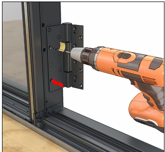
Figure 30 Use a tape flag to drill to the correct depth.
