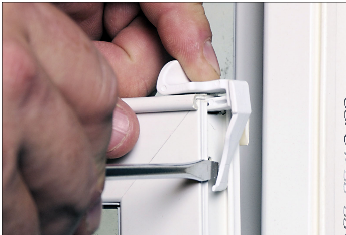
Figure 1: Remove old tilt latch with a screwdriver.
