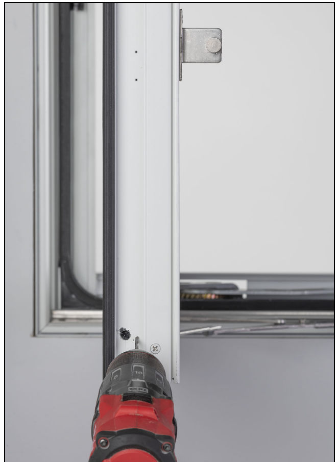
Figure 3 Predrill sash
