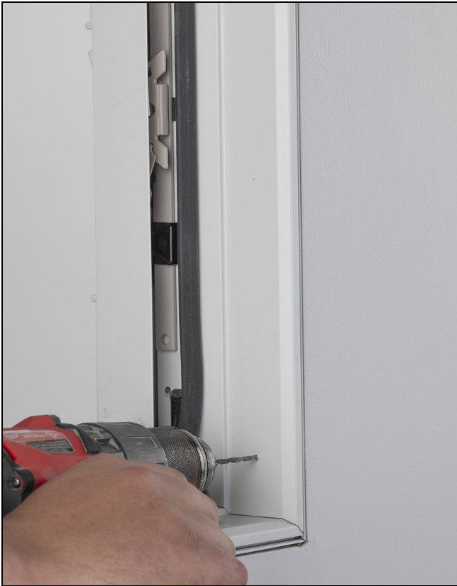
Figure 4 Predrill frame locations
