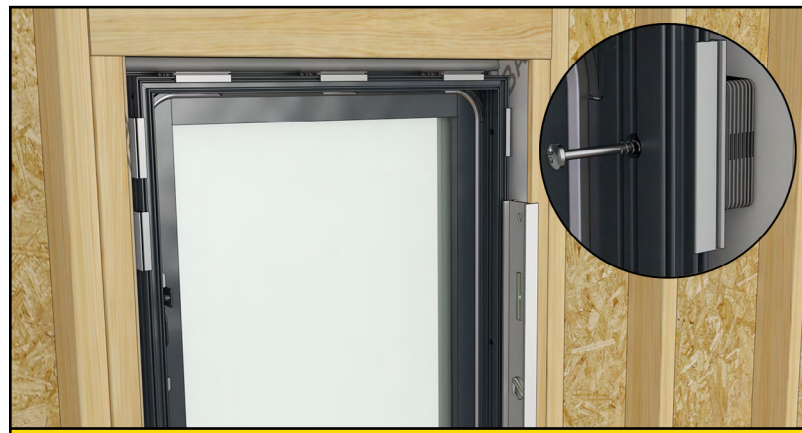
STEP 6 Plumb one jamb and fasten the top corner..
